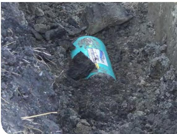
Automatic water control valve (in place).
