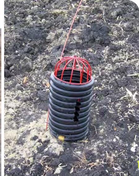
(L) Demonstration site: Slotted riser and gravel inlet. (R) Slotted-raisd inlet. Kandiyohi County, MN.
