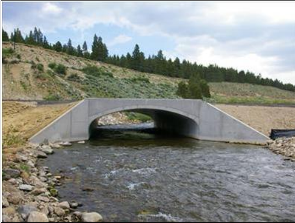
Figure 15: Photograph and Schematic of Pre-Cast Bottomless Culvert.
