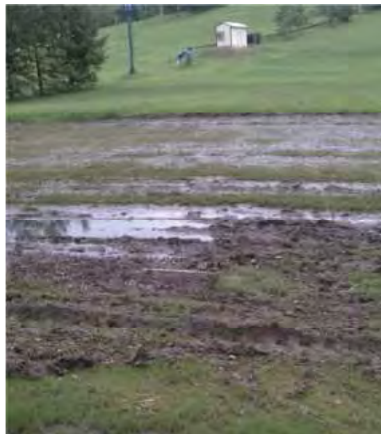
Figure 3. Typically Muddy Conditions at Base of Slope Due to High Water Table (Photo: HR Green)
