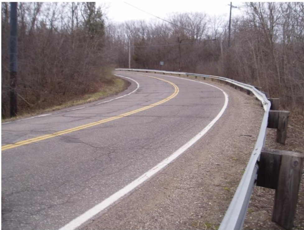
Project Area facing east.
