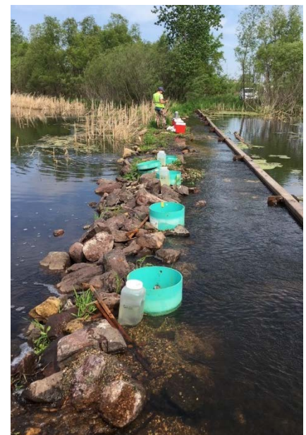
Kohlman Basin permeable weir system with CC17 test cells. Photo Credit: Keith Pilgrim
