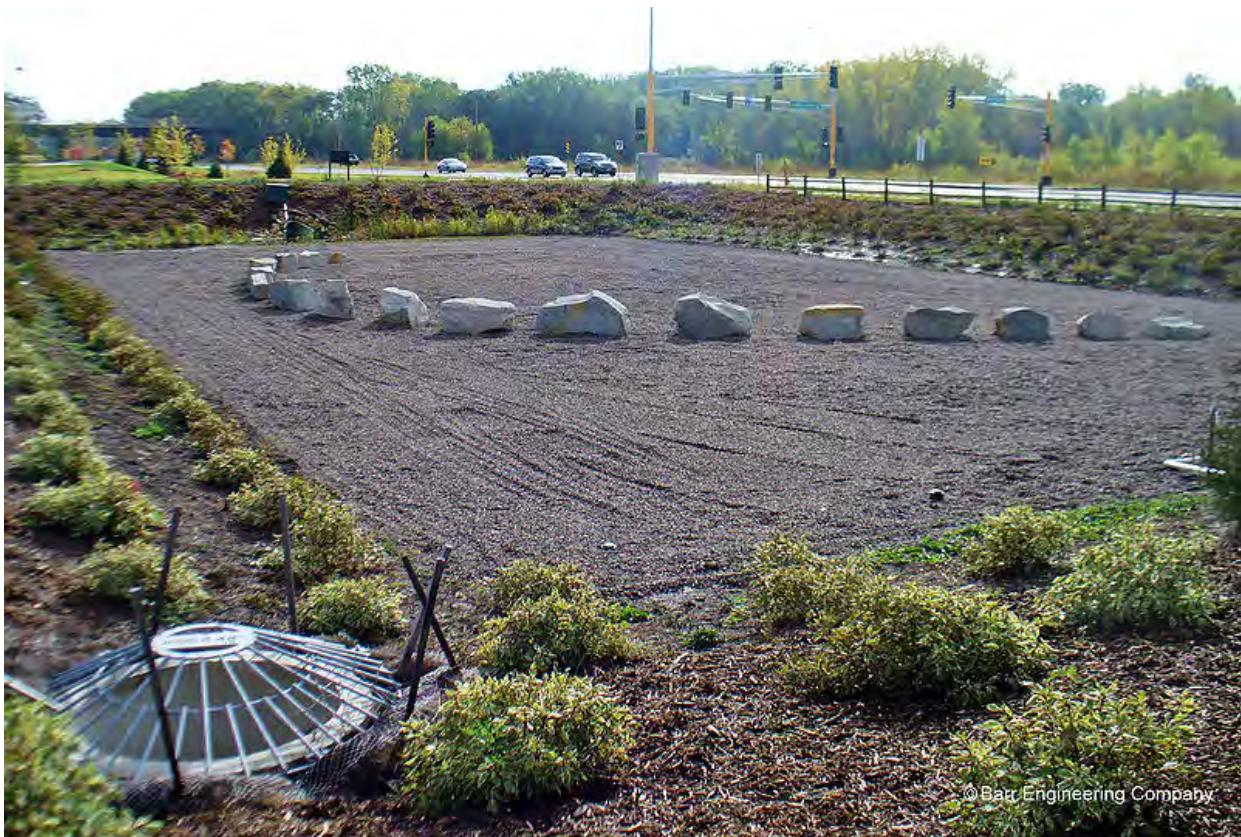
Figure 5: Iron Enhanced Sand Filter Basin
