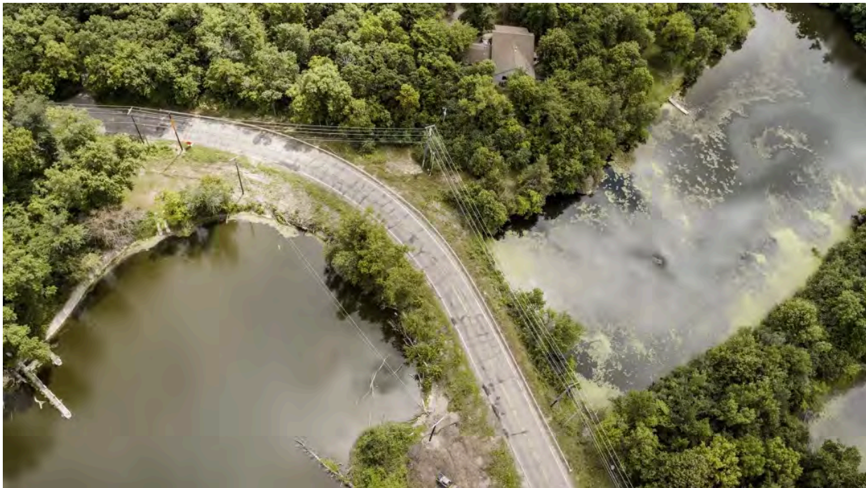
The new bridge, built by Washington County and South Washington Watershed District, allows Grey Cloud Slough to flow freely through the area for the first time in 50
