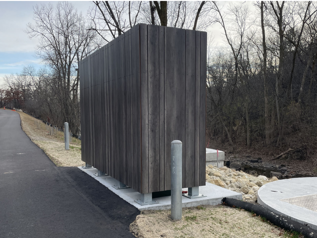
Screen Wall Side View (facing south)
