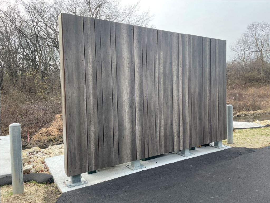
Screen Wall Front View (facing east)
