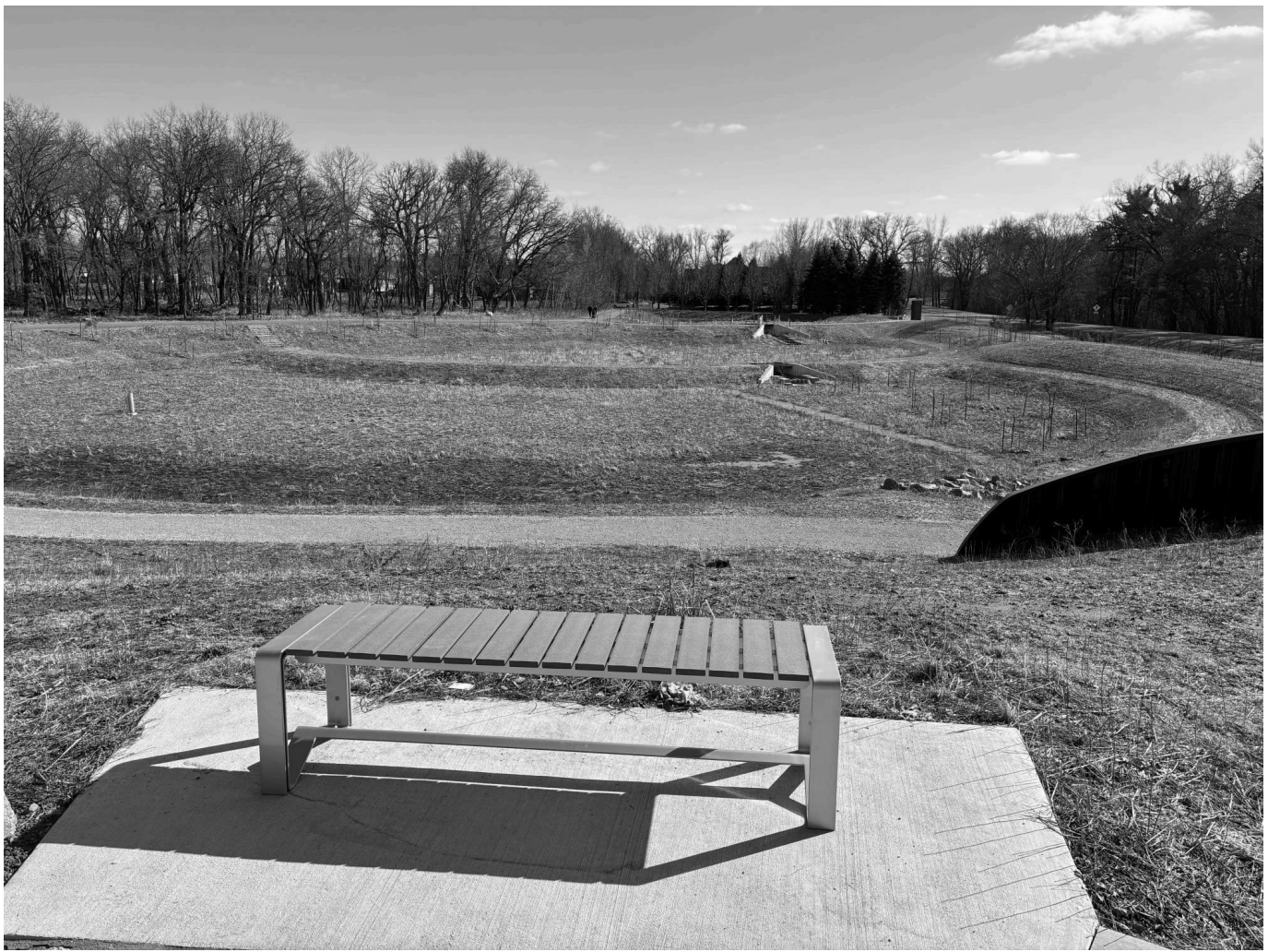
An early April view clearly shows the three interconnected infiltration basins at Hasenbank Park. (Image by Doug Schultz)
